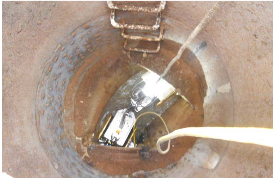
Figure 7. SewerVUE Surveyor robot operating at Harvard Gulch, Denver, CO.
