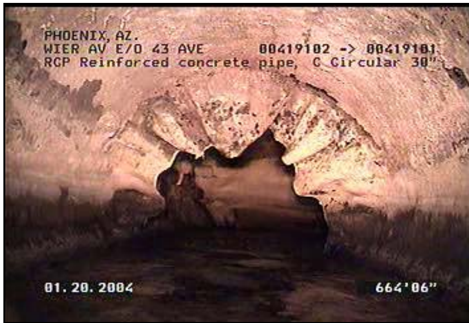
Figure 2. Detached liner
