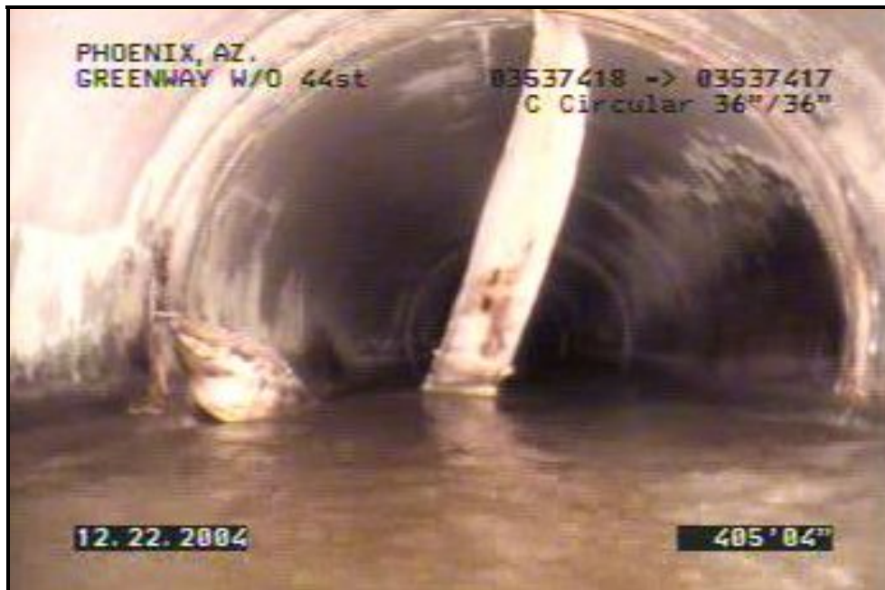
Figure 3. Detached weldstrip
