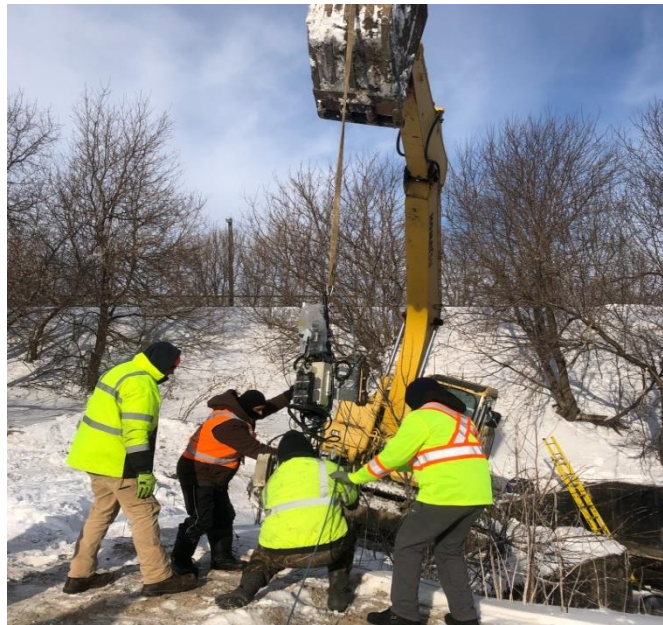
Figure 4: Surveyor deployment in the RC pipe
