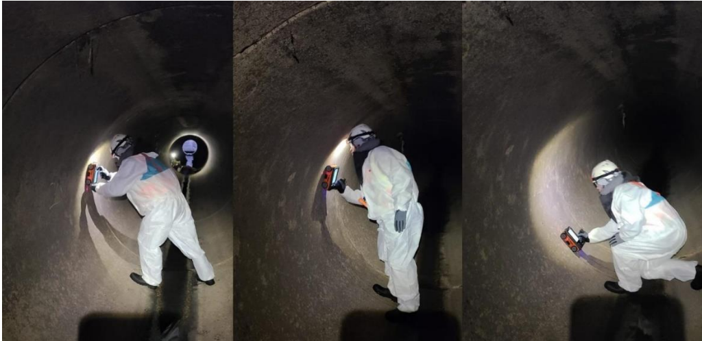
Figure 1. SV Technician during inspection
