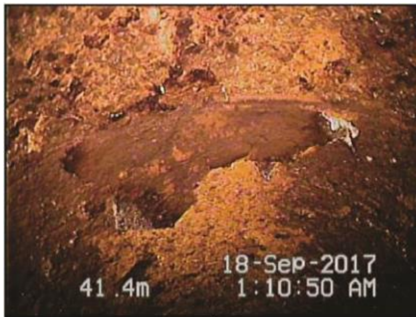
Figure 8 - CCTV image from the Maribyrnong Main showing spalling and visible aggregate
