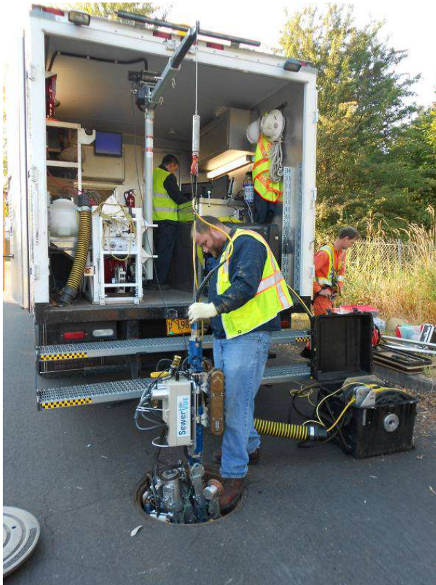
Figure 3: Insertion of the SewerVUE Surveyor robot at manhole 28-303.
