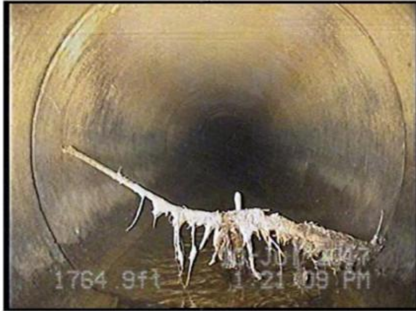
Figure 5 - CCTV image showing a significant intruding root
