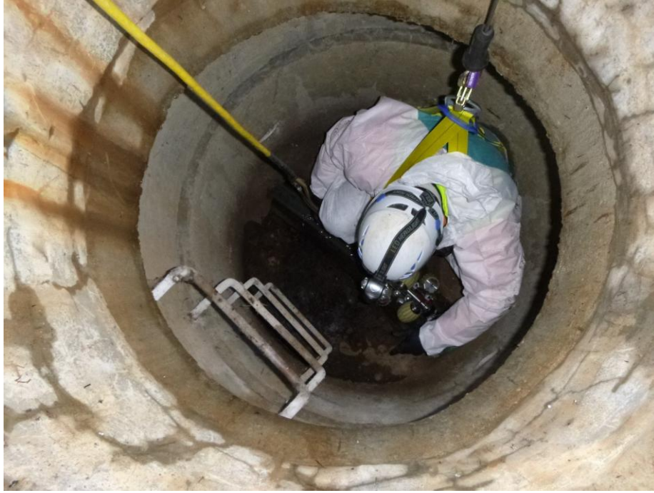
Figure 3 - A SewerVUE technician places the ACPS into the Harbourgreene line.
