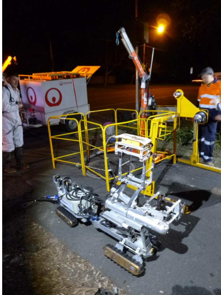
Figure 1 - The SewerVUE Surveyor robot on-site in Melbourne, Australia
